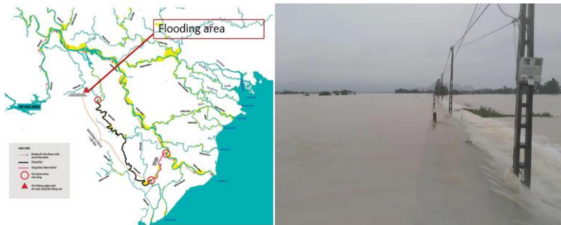
Figure 1.9. Floodplain position and overflow through the dyke on Bui river
